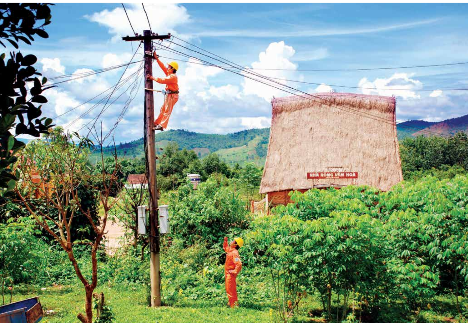
EVN's workers repaired and renovated the power grid in Central Highlands
